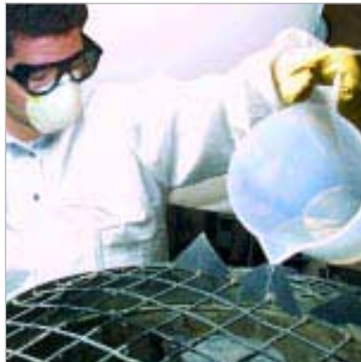
3. Mixture too dry: gradually add up to 30 ml of water per 25 kg of KALCRET.
