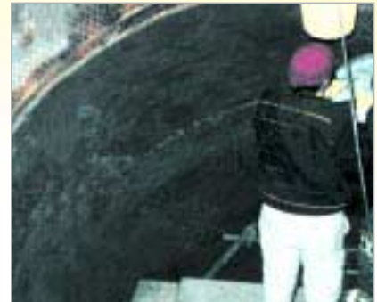
Raw meal duct in a cement plant.
