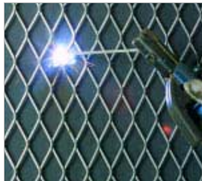
Welding of metal wire mesh: spacing approx. 250 mm.
