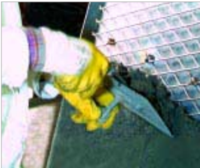
1. Prepare compound to be trowelled as specified.
