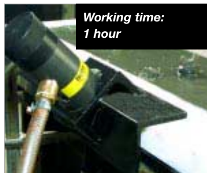
4. Use external vibrator for compacting.
