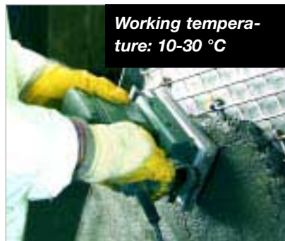
2. Apply sufficient KALCRET and compact it.
