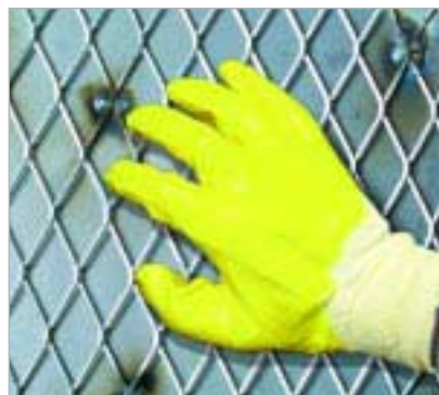
Stiff and firm fastening, distance to surface to be lined approx. 5 mm.
