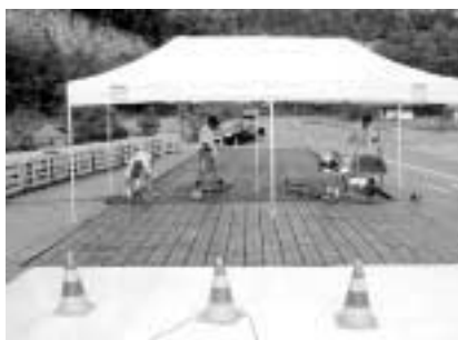
Installation of the test track with ABRESIST fused cast basalt.
