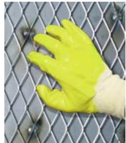
Stiff and firm fastening, distance to surface to be lined approx. 5 mm.
