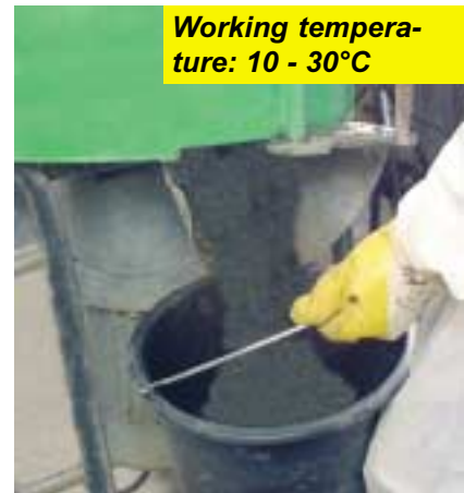
Prepare cast compound as specified.
