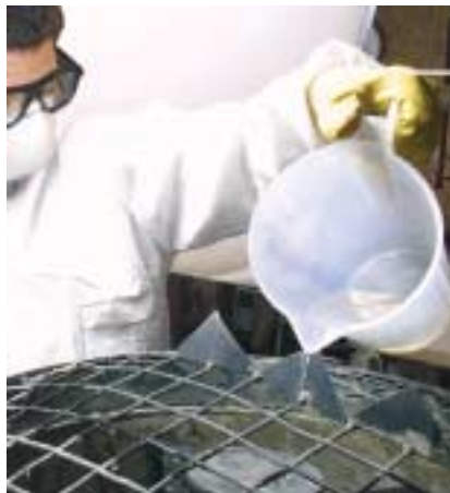
Mixture too dry: gradually add up to 30 ml of water per 25 kg of KALCRET.
