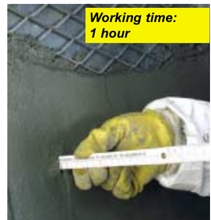
Check thickness and make it uniform, if necessary.
