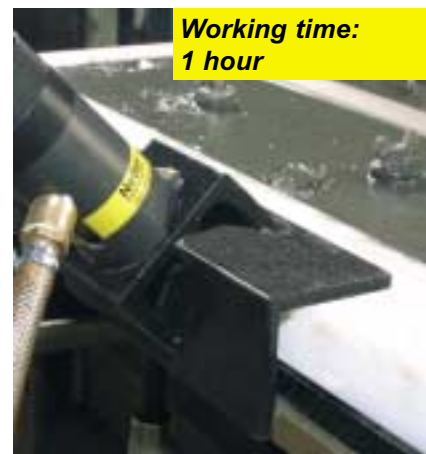
Use external vibrator for compacting.
