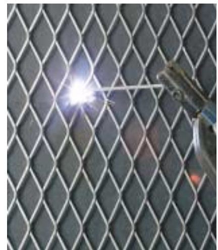
Welding of metal wire mesh: spacing approx. 250 mm.
