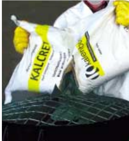
KALCRET and water to be mixed as specified in the working instructions.
