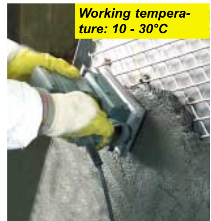
Apply sufficient KALCRET and compact it.
