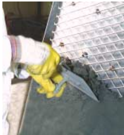
Prepare compound to be trowelled as specified.
